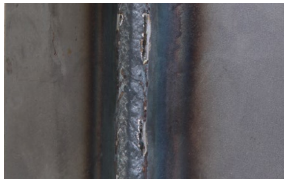
Root welding in PA position with an air gap and without weld pool backing
